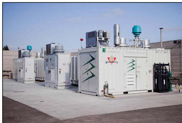
Photo 4: Many fuel cells, like these FuelCell Energy units, can run on natural gas or biogas
